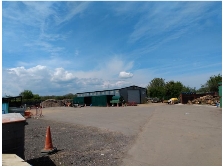
Fig. 1 – Existing workshop building
