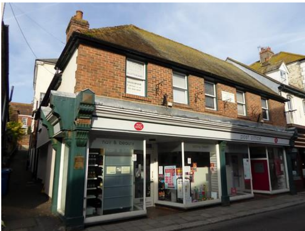
Figure 3 – shopfront prior to unauthorised work
