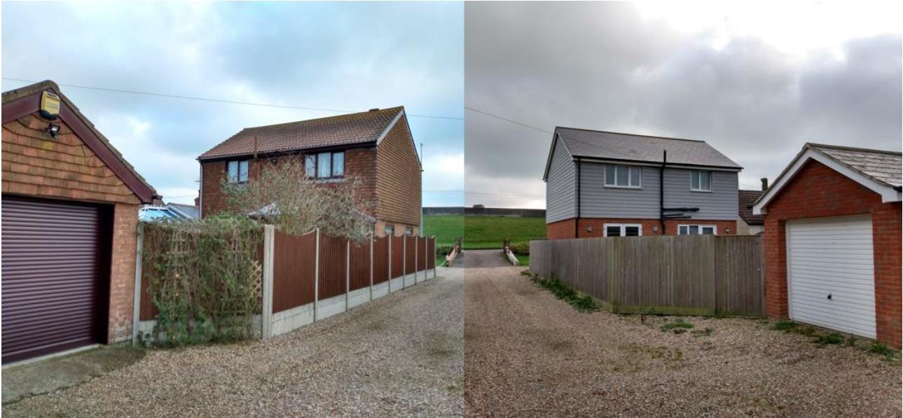
Photo 4: Rear of 1 and 2 Willop Close
